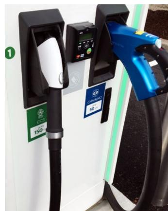
ABB charging stations on Electrify America's network accommodate both CHAdeMO and CCS-1 compliant vehicles in multiple power levels.
